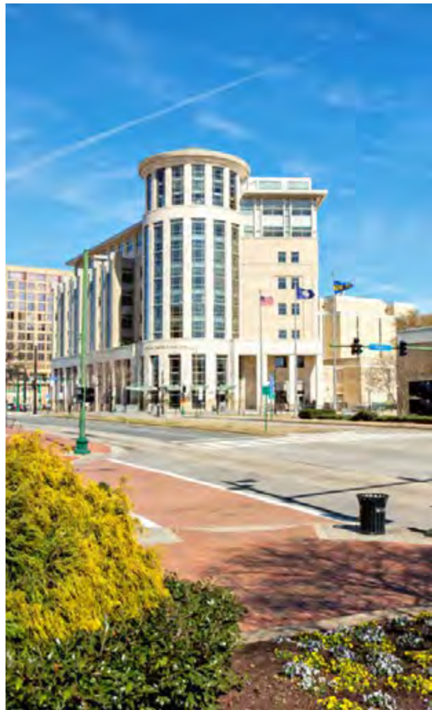
NORFOLK CONSOLIDATED COURTS: Walsh is constructing this 315,000 SF facility that consolidates the Operations of the Circuit Court, General District Court, and Juvenile and Domestic Relations Court.
